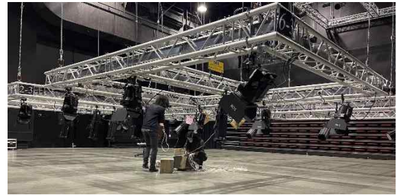
Figure 3. The space has eight individually height-adjustable truss sections. The photo is taken during tests of a mock-up loudspeaker arrangement.
